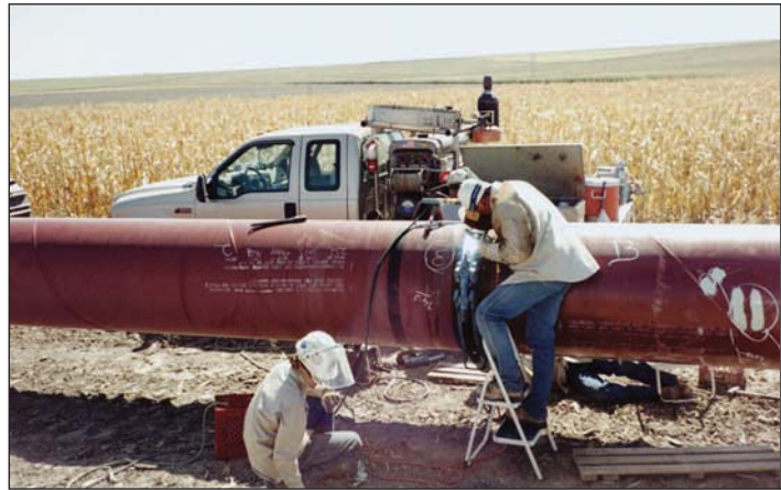
Cross-country pipe welding.
